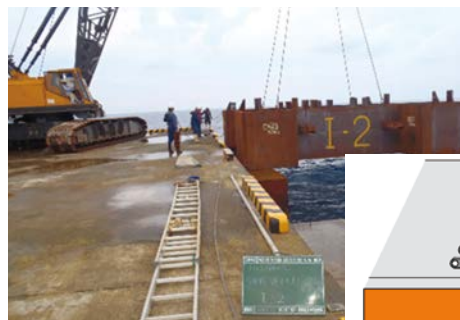
Installation of steel formwork
