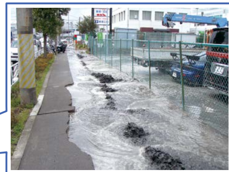
Liquefaction caused by the Great East Japan Earthquake (March 11, 2011) • Sand and groundwater is gushing out of the crack in the road.
