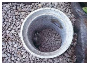
Infiltration inlet
