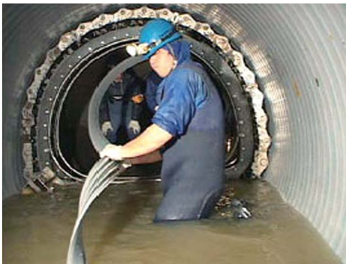
Reconstruction work inside a circular-shaped sewer
