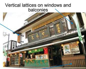
Air conditioning units camouflaged to preserve the historic appearance
