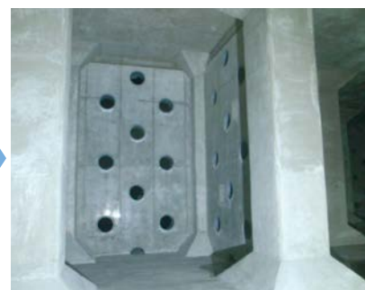
After seismic reinforcement (installation of quake resistant walls)
