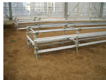
Frame is easily put together using pipes available at retail stores
