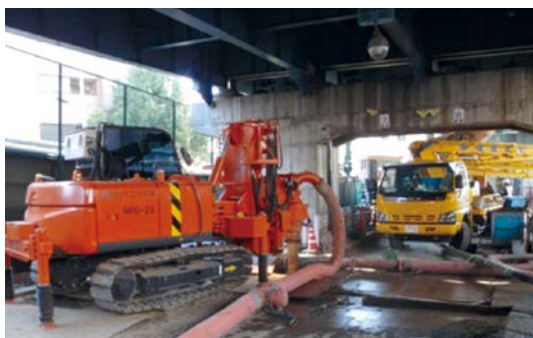
Installation of additional piles
