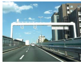
Fixed cameras on an expressway
