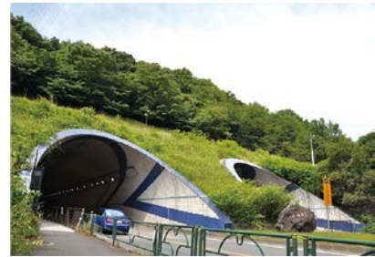
Oyamadairi Tunnel (completed in 1990)
