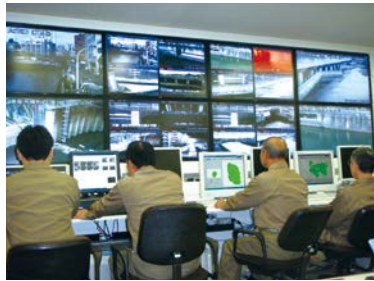
Monitoring room (During flood control activities)
