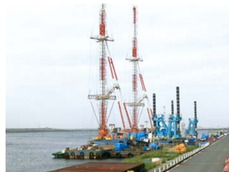
Drain placement ship
