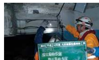
Repairing by electric anticorrosion
