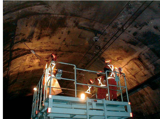
Inspection by sounding concrete
