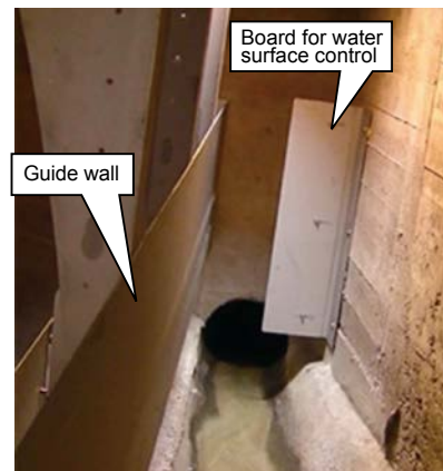
Installation of water surface control device (case of Germany)
