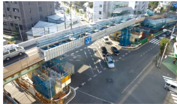
Main girder replacement
