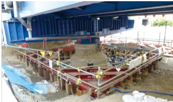
Reinforcement of footing
