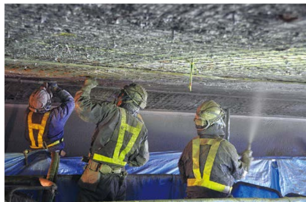
Workers repair a deteriorated concrete surface by spraying (cut-and-cover tunnel).
