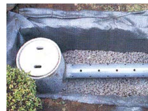
Infiltration trench
