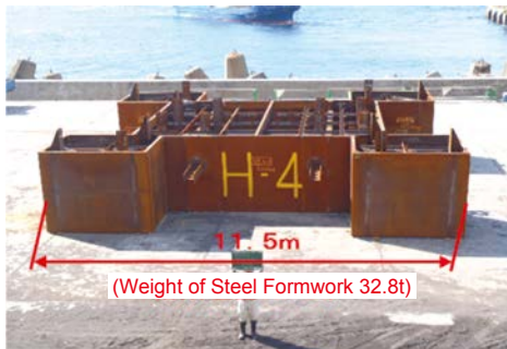
Completed assembly of steel formwork
