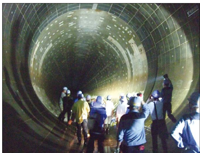
Wada-Yayoi Trunk Sewer (Inspection tour after completion)
