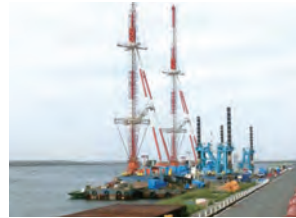
Drain placement ship ※ 2
