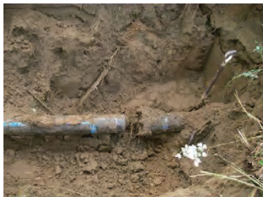
<An uncoupled joint that was not seismically designed (Niigata Prefecture)> (Source: Ministry of Health, Labour and Welfare) ※ 1
