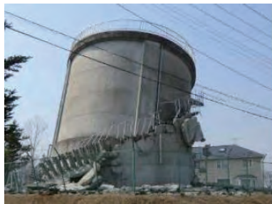
<A water tower that tilted from an aftershock of the Great East Japan Earthquake (Iwate Prefecture)> (Sources: Ministry of Health, Labour and Welfare / Japan Water Works Association) ※ 2
