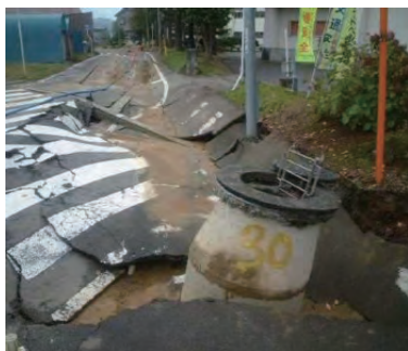
Niigata Prefecture Chuetsu Earthquake Oct. 23, 2004 (Tokamachi, Niigata Prefecture) ※ 1
