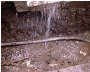
Leak from a lead water pipe ※ 1
