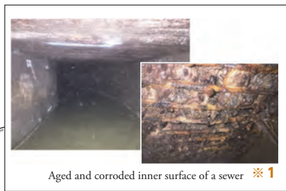
Sewer before reconstruction ※2
