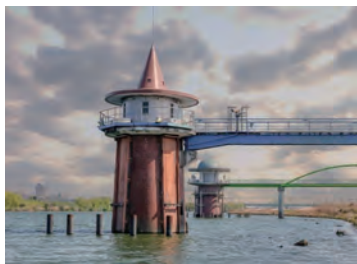
Intake tower at the Kanamachi Purification Plant ※1
