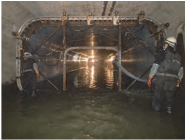
Rehabilitation work using this method ※ 3
