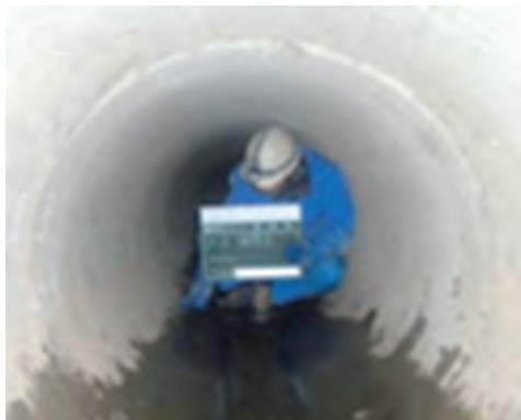
Internal inspection of water mains by interrupting water supply ※ 1
