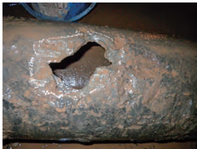
Leak from a corroded cast iron pipe ※ 2
