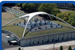
Making TMG-Owned Buildings Greener ..... p09
