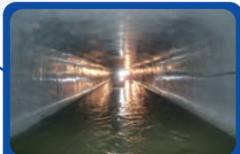
Sewer Rehabilitation Method ..... p39
