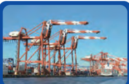
Constructing Port Facilities on Soft Ground ..... p23
